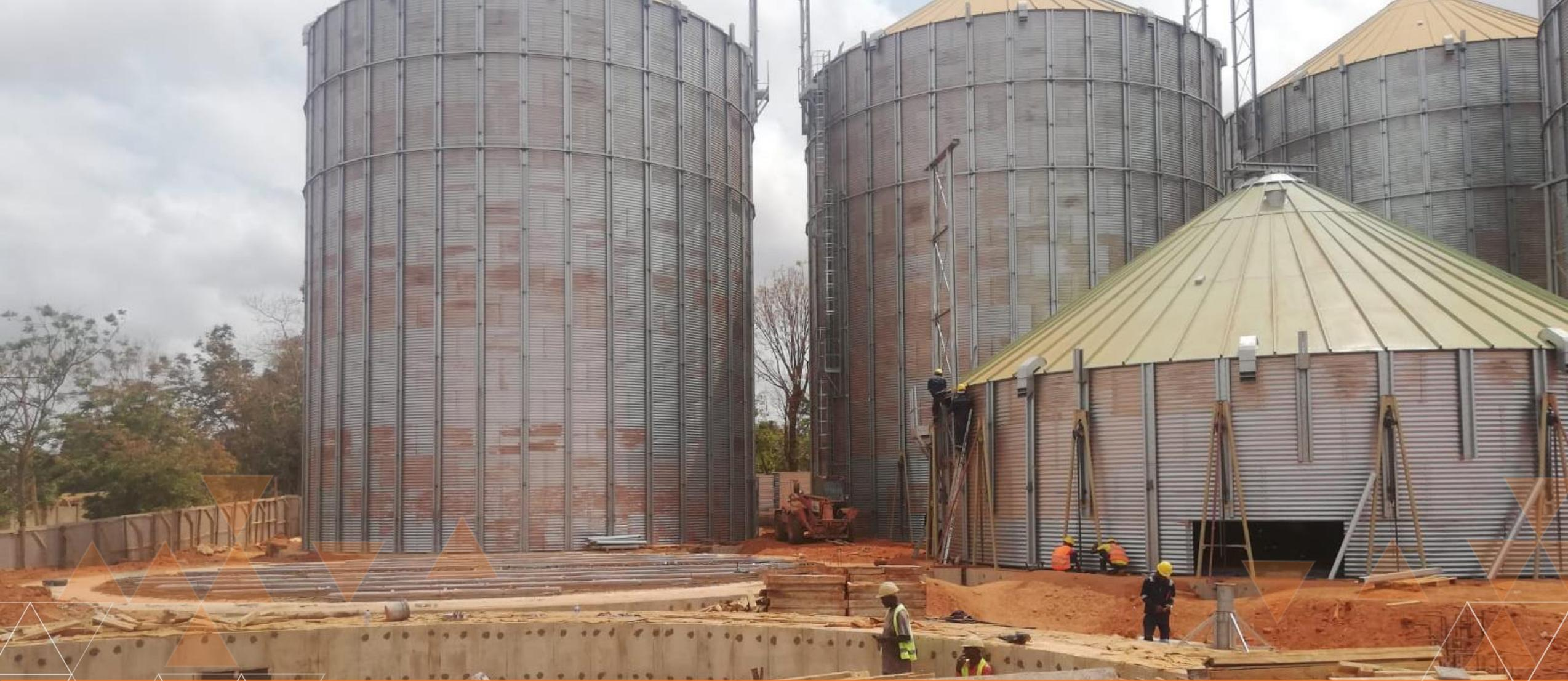
In parallel with the installation of roofs and sheathing, we conduct further foundation works for further silos, flat warehouses and other parts of warehouse complexes.
